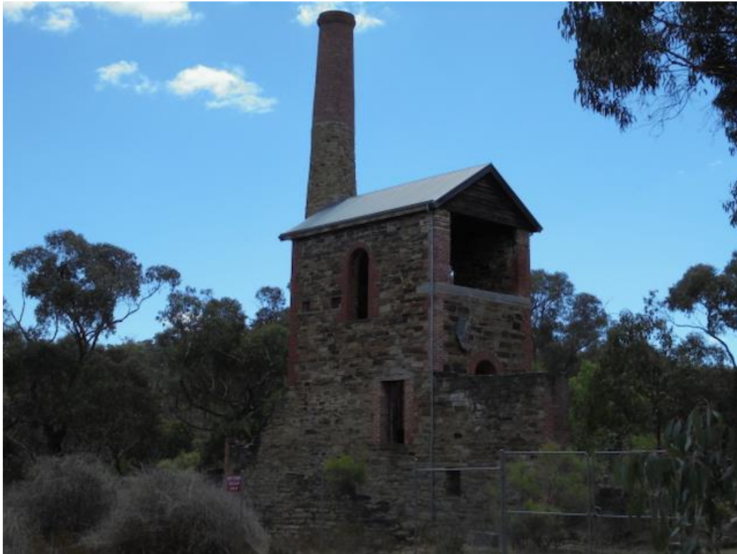
Duke of Cornwall Engine House, Fryerstown.
