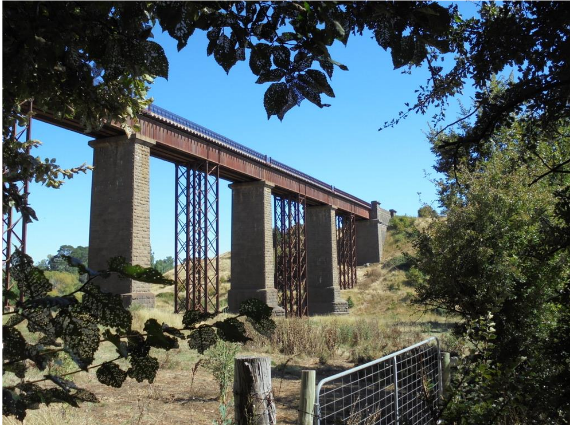
Taradale Railway viaduct (1862).
