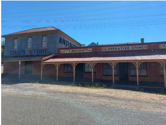
Old stores – dating from 1854 on Templeton St
