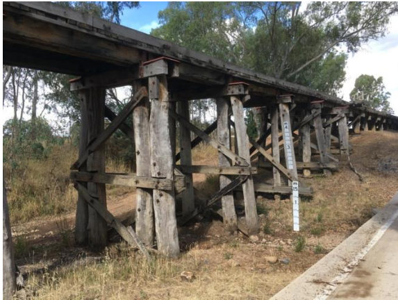
Trestle bridge over Muckleford Creek.
